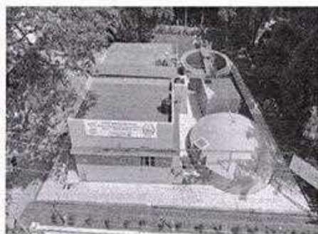
360 KLD STP at General Hospital, Thrissur
