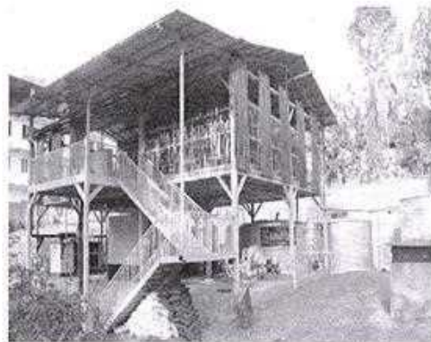
1 MLD STP at Kozhikode medical College
